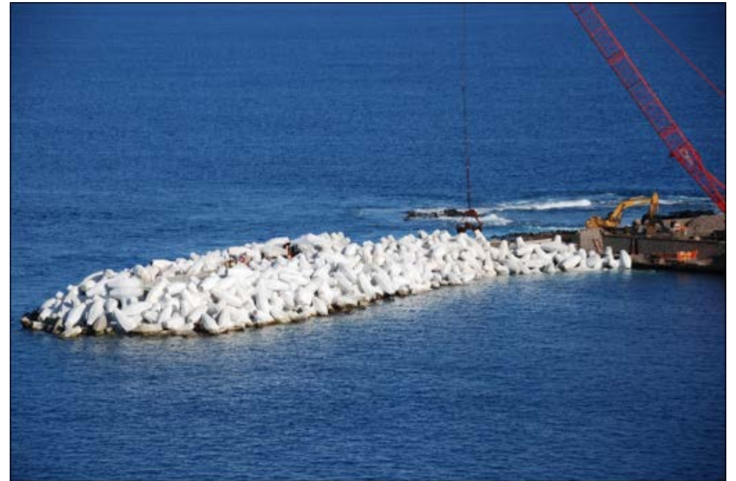
Kaumalapau Harbor Breakwater Repair Project
